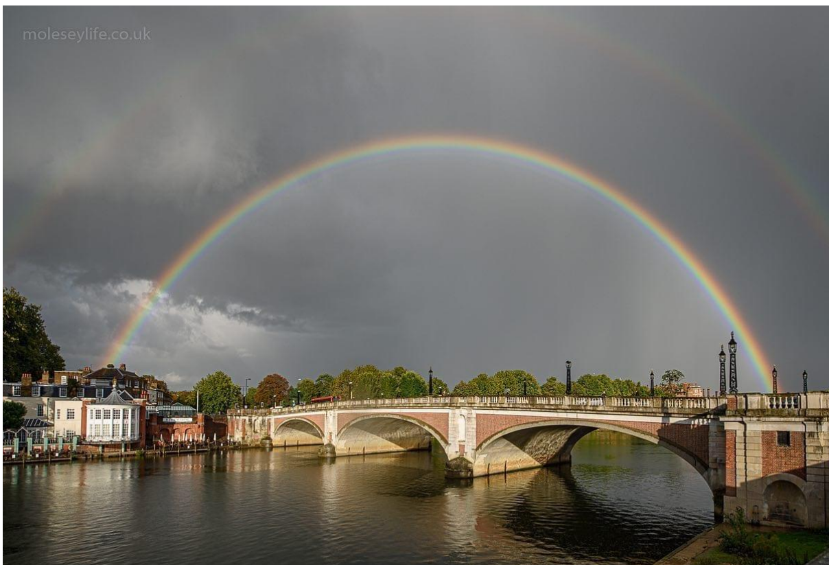
16. Upstream, the strong light catches the underside of arches and the lamp standards.
