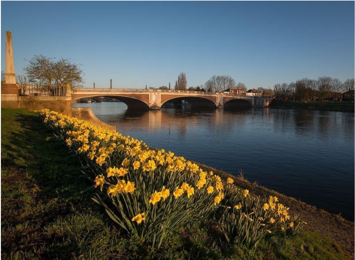
17. Downstream, from Cigarette Island Park, a simple structure that gives a serene setting to the Palace opposite.
