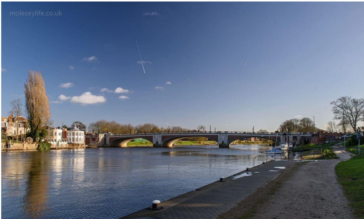
13. Upstream, the simplicity of the three arches is complimented by the horizontality of the parapet, only broken by the verticality of the lamp standards.
