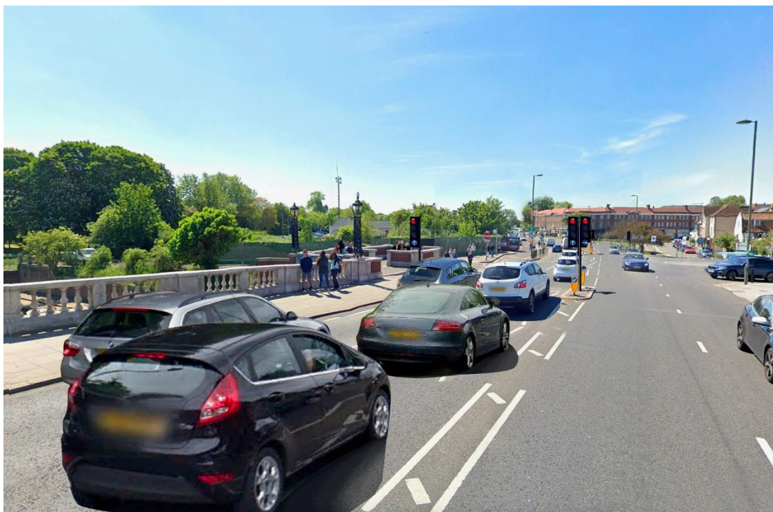
3 & 4. Note how the vertical traffic lights take the emphasis away from the elegant lamp standards on the bridge and split uninterrupted view south (see note to Fig. 1 on the design, dimensions & context)
