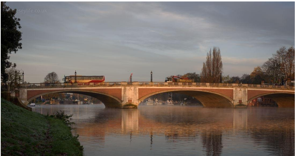
18. Downstream, from Cigarette Island Park, the traffic signals will be sites in the far-left corner just after the lamp standard.
